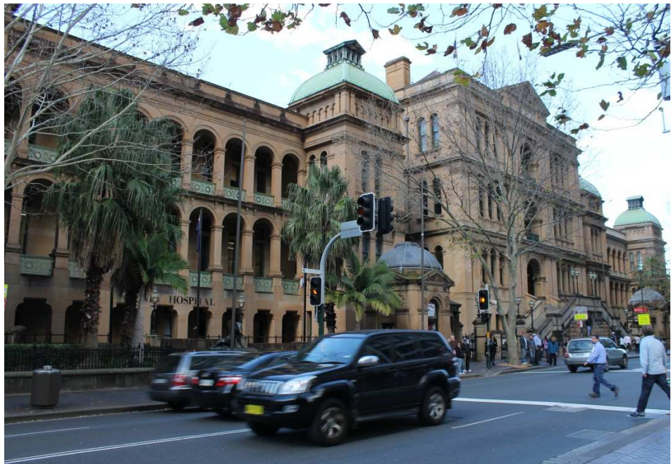
Sydney Hospital group of buildings
