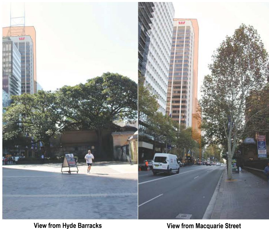
Figure 58 – Views of building envelope in skyline Source: Hassell
